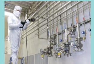
Constructing supply piping for high purity gases
