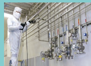
Constructing supply piping for high purity gases
